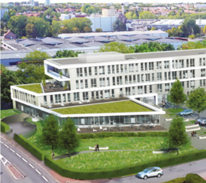
Business Office – bât. A – Marcq-en-Barœuil (59)
