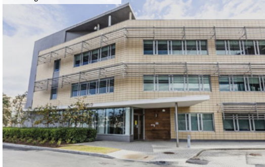
Building 8 – Dublin – Irlande
