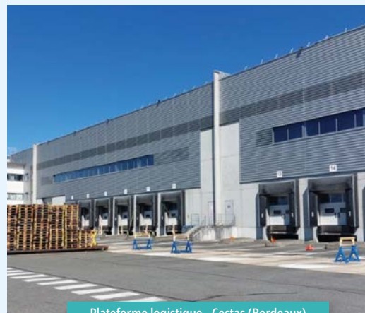
Plateforme logistique - Cestas (Bordeaux)
